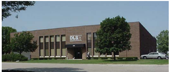
D.L.S.'s 30,000 sq. ft. headquarters in Wheeling, Illinois
